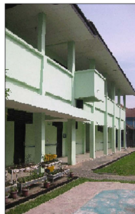
Figure 1. Image of the YPAC Building Medan 2015
